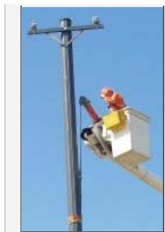
Pultrusion specialist Bedford Reinforced Plastics (Bedford, Pa.) featured in its booth a utility pole that it manufactures for customer Duratel (Chicago, Ill.). Source: Bedford Reinforced Plastics
